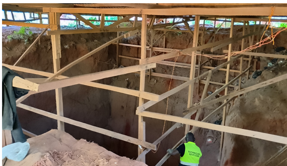
◀ Mining pit in Kamilombe protected by a timber-framed structure.
