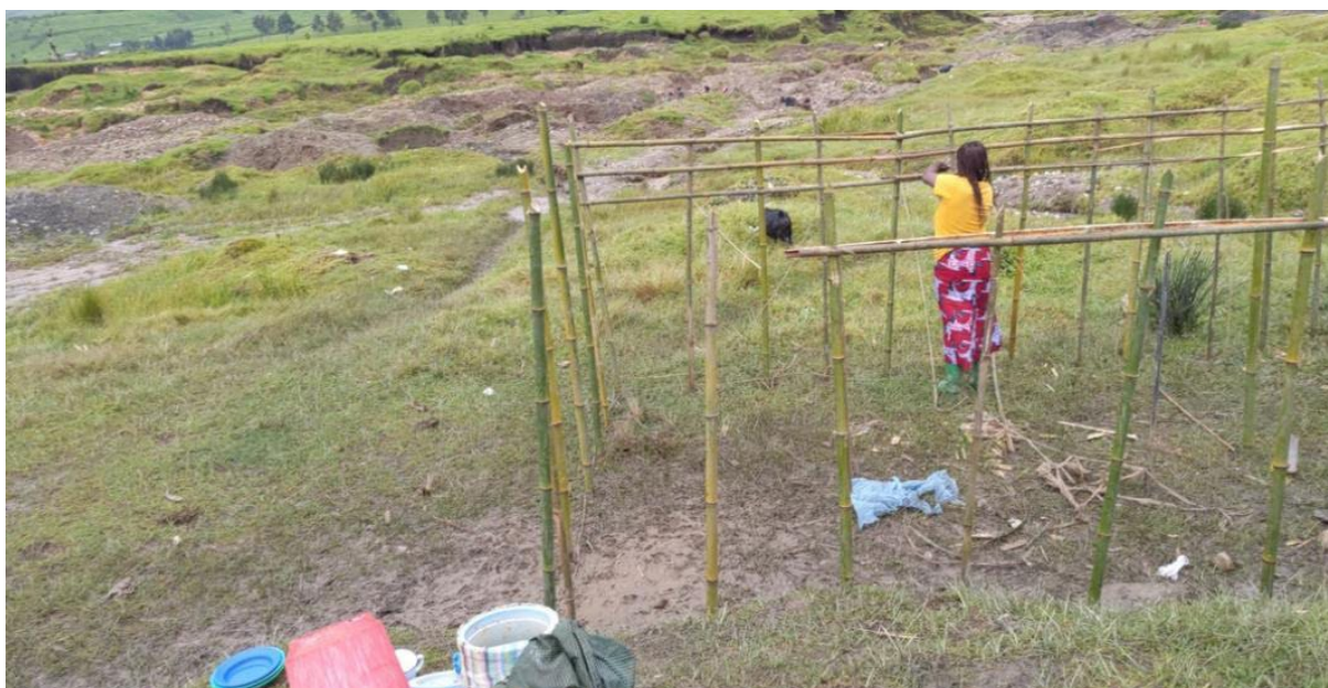
Construction of a makeshift restaurant on a mine site, Numbi.
