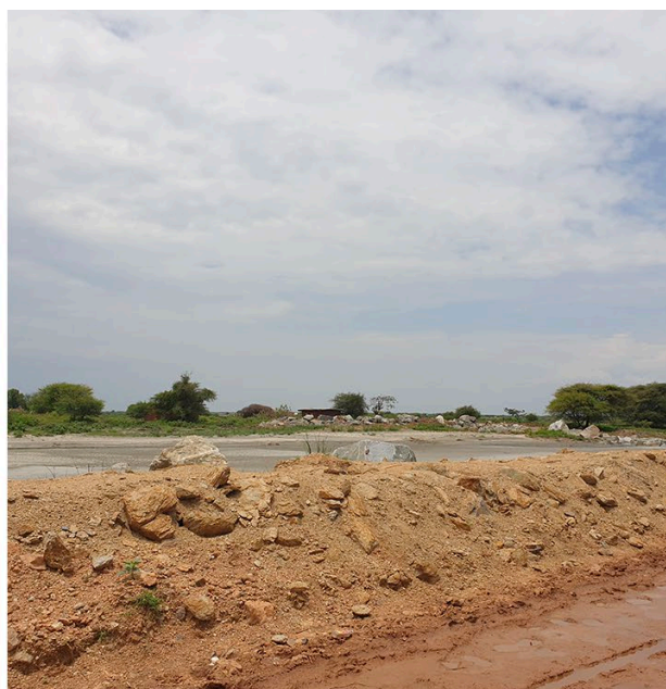
▲ Figure 2.4 Examples of small containment structures that were built in Ng'wangh'olo to limit the spread of the tailings slurry, as observed in February 2023 (Photo: IPIS, 2023)
