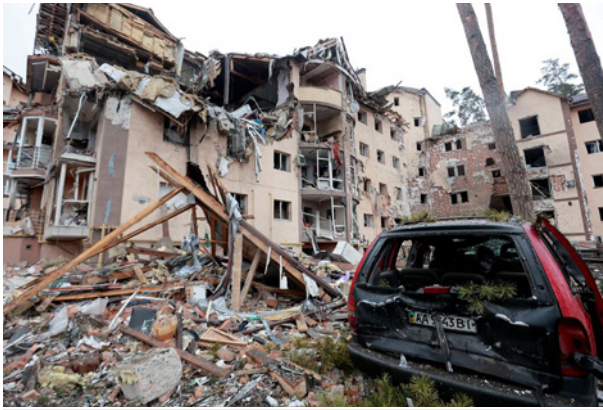
Residential building destroyed by shelling in Irpin, Ukraine, 2 March 2022 (Photo: Serhii Nuzhnenko, Reuters)
