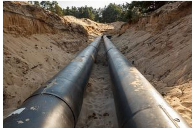
Figure 5 Example of a pipeline in its trenches
