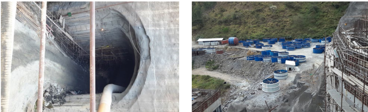
Figure 5: Underground Blasting to Create a river diversion (L). Channel and Turbines (R), causing enormous vibrations that are felt a long way from the site
