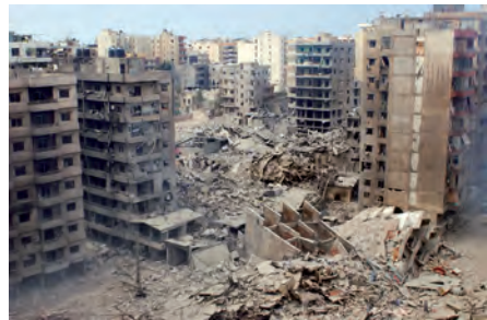
Damaged buildings in Haret Hreik, Beirut, Lebanon, following the conflict with Israel in July of 2006. GMES services for Security applications can provide, inter alia, support to EU External Action such as peacekeeping operations and post-conflict reconstruction missions (Credits: UN-OHCHR).
