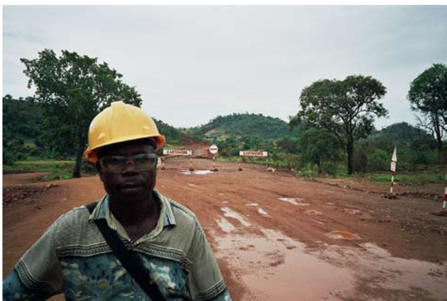
Within the TFMining concession, major road works continue. (Photo IPIS)
